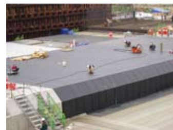
Worksite of Incheon International Airport
