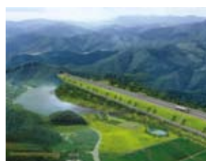
Lake/Non-point Purification Facility
