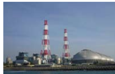
Taiwan Hsinta Plant Unit 1, 2, desulfurization, electric precipitator, ash handling facility
