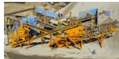
Worksite of Goyang city, Gyeonggi-do
