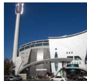
Goyang-si Environmental Energy Facility
