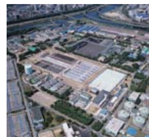
Jungrang Sewage Treatment Plant
