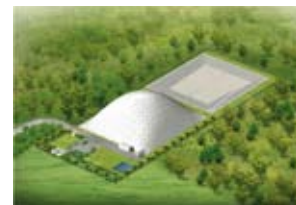
Appointed waste landfill using air dome technology
