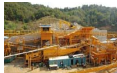
Worksite of Hwaseong city, Gyeonggi-do
