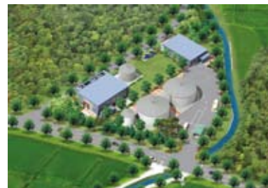
Wanju-gun energization worksite
