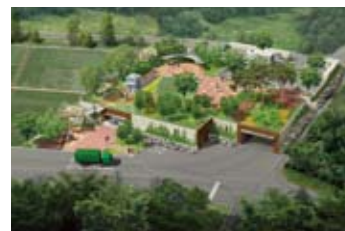
Jungnang-gu Material recovery facility
