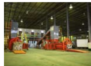
MSW pre-treatment facility in Vladivostok, Russia
