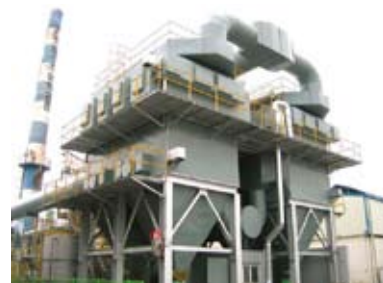
HI-FILTER installation site
