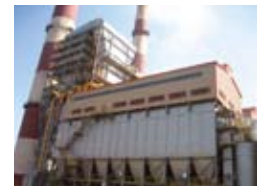
Gwangyang Iron Co., Electric precipitator
