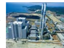
Electrical Precipitator for Yeongheung Thermal Units 1 and 2
