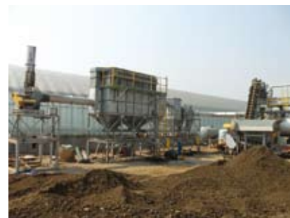
LPP worksite in Paju
