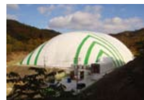
Complete view of air-dome type landfill
