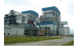
Taishan Power Plant in China
