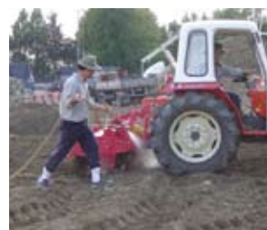
Spraying microbial substance for purification of polluted soil
