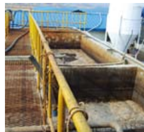
G Farm's Livestock Excretion Treatment Facility
