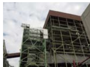
Boryong Thermal Power denitrification facility
