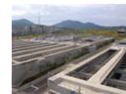
Paju LCD Industrial Complex Wastewater Treatment Plant
