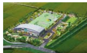
Jeongnam Sewage Treatment Plant
