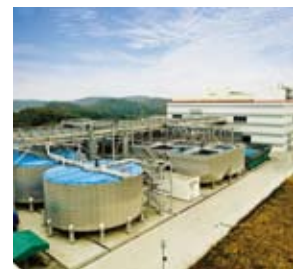
LCD P7 Environmental Facility
