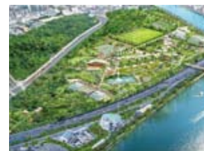
Busan Suyeong Bay Sewage Treatment
