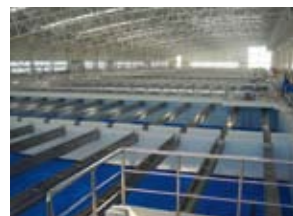
Harbin 2 nd Water Purification Center, China
