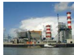
Haripur Thermal Power Plant
