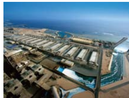
Shuaibah Desalination Plant, Saudi Arabia
