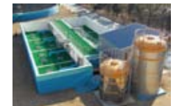
Daegu Dalseong Wastewater Treatment Plant, Advanced Sewage/Wastewater Treatment
