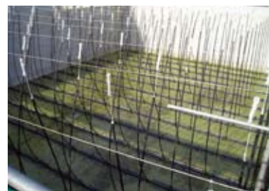
Namyangju Sewage Treatment Plant CSBR Site
