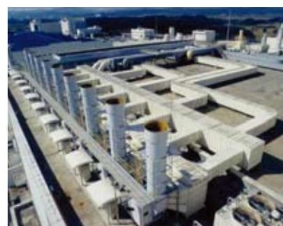
Cheongju Hynix semi-conductor scrubber system
