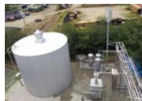
Namyangju, Jingeon sewage treatment plant
