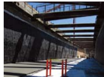
Worksite of Bart in San Francisco USA
