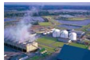
Ratchaburi Water Treatment Plant, Thailand (271,440m 3 /day)
