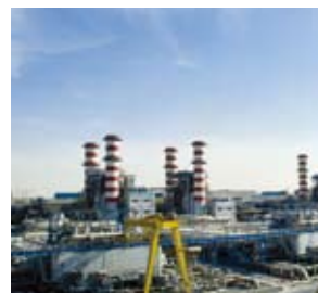
Jebel Ali M Combined Cycle Power Plant, UAE
